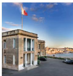
Cover: Sir Paul Boffa Hospital, former King George V (KGV) Hospital, is not only a military building but it was initially opened in 1922 as a memorial to the men of the Merchant Navy who died in World War I. The building was severely damaged in 1942 during World War II, and although there had been a temporary halt due to air raid bombardment, the hospital services were never interrupted. The memorial was then rebuilt in 1948 under the premiership of Paul Boffa and renamed Sir Paul Boffa Hospital in 1976. This building has been in existence for over 50 years, and out of all the naval hospitals in Malta to date it is only Zammit Clapp Hospital and Boffa Hospital that still maintain a medical function.
